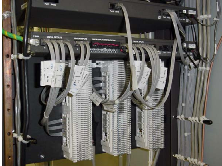
FIGURE 9-19 EXAMPLE OF CABLE LABELING
